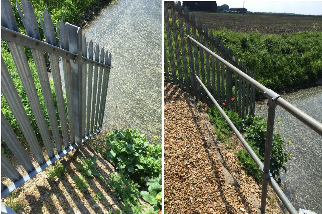
Figure 2 Typical environment where level sensor will need to be installed
